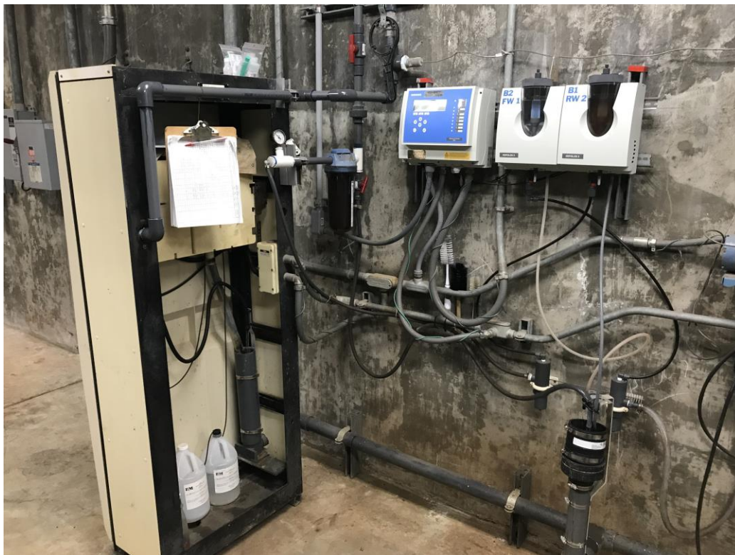
Back of the Obsolete Chlorine Analyzer (Left); Type of Replacement Analyzer (Right)
