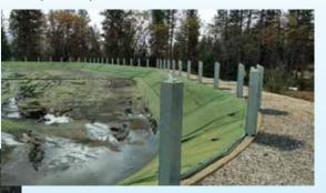
Reservoir B is currently an in-ground storage tank with an aging liner and "floating" cover.
