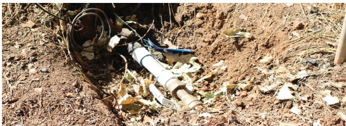
Example of a removed meter replaced with a pipe and shut off valve.
