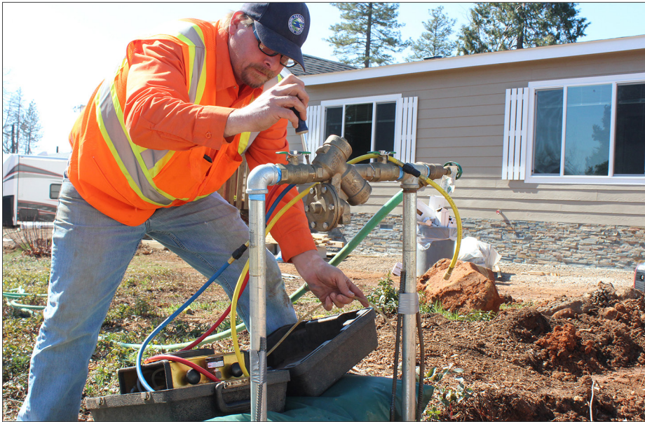
PID employee Marc Beckham tests the operation of a backflow device.
