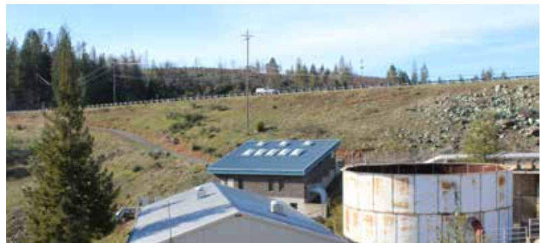
PID continues work to identify retrofit options for Magalia Dam, seen here from below the dam, near the PID Treatment Plant.
